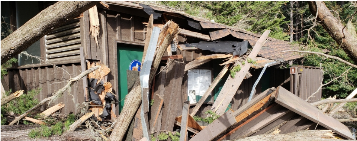
Damage at Julia Pfeiffer Burns State Park due to recent storms.
